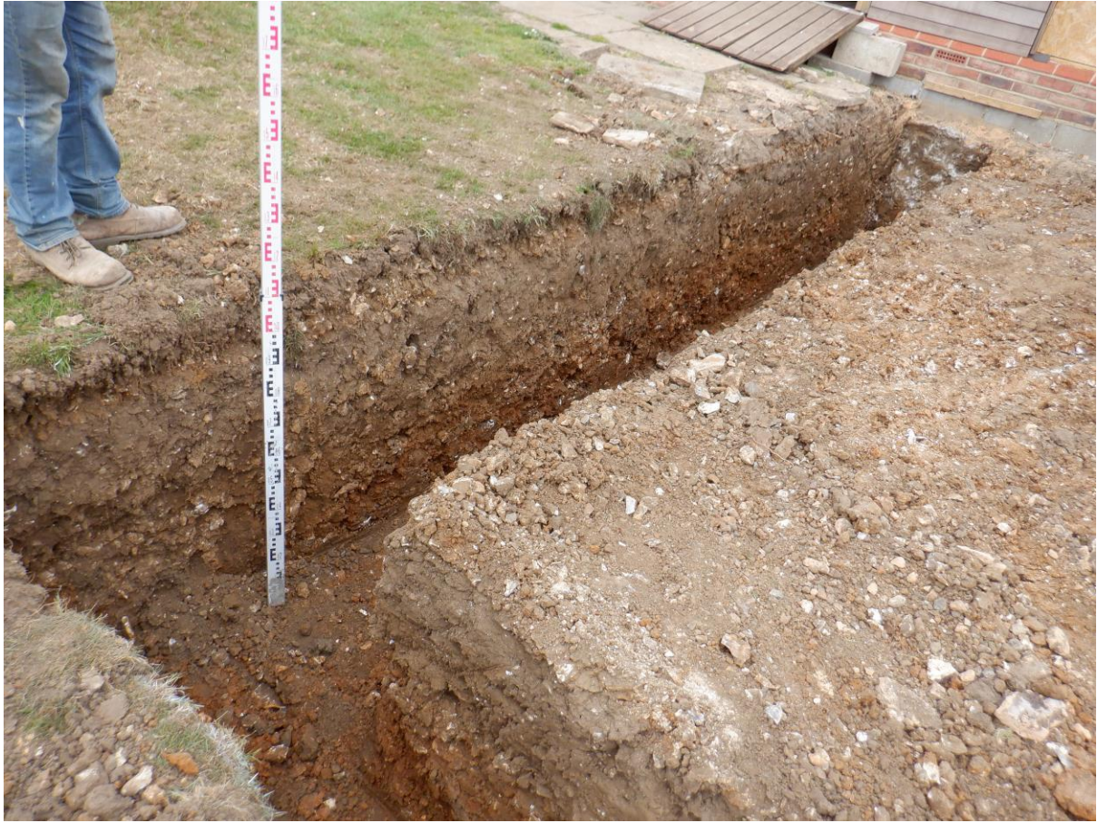
Plate 3. View of completed single storey extension foundations (looking NNE)
