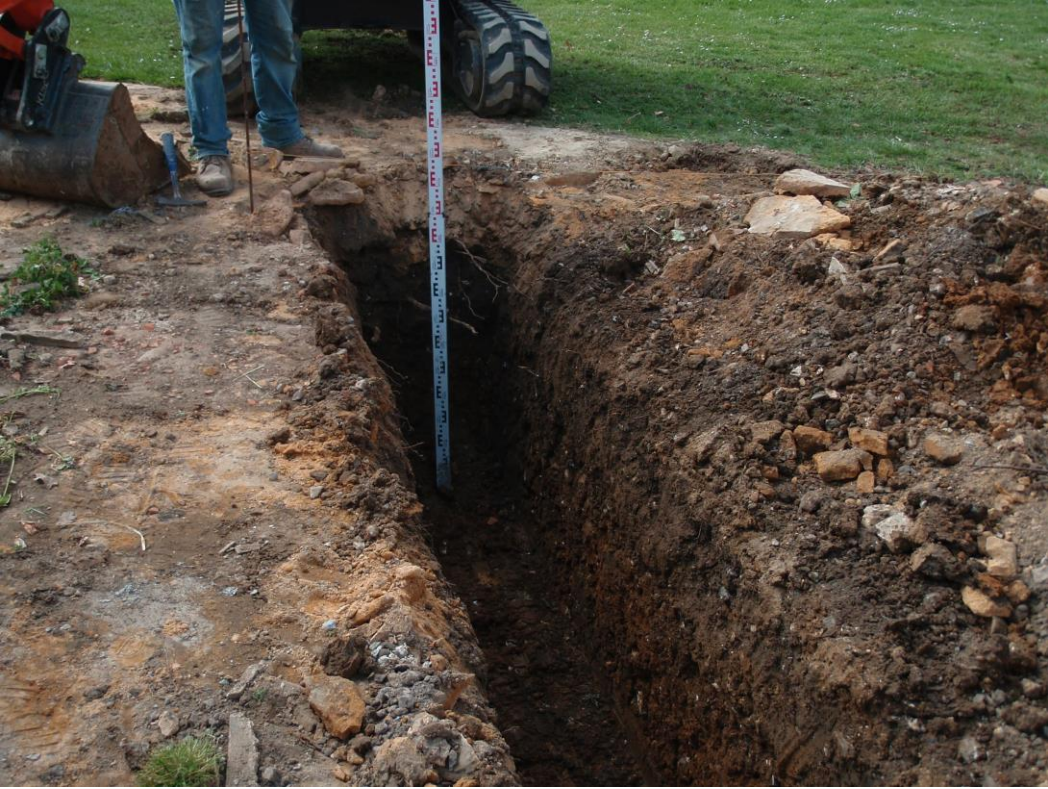
Plate 1. View of the site – single storey extension foundations (looking SW)
