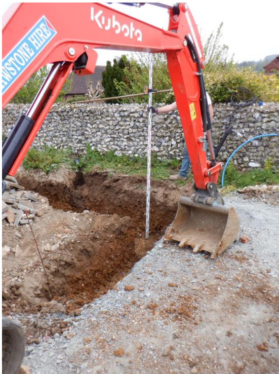
Plate 4. View of garage foundation trenches (looking NNE)
