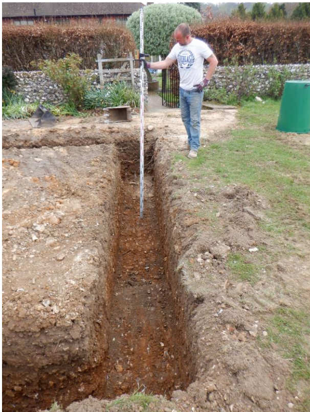
Plate 6. Completed garage foundation trenches (looking E)
