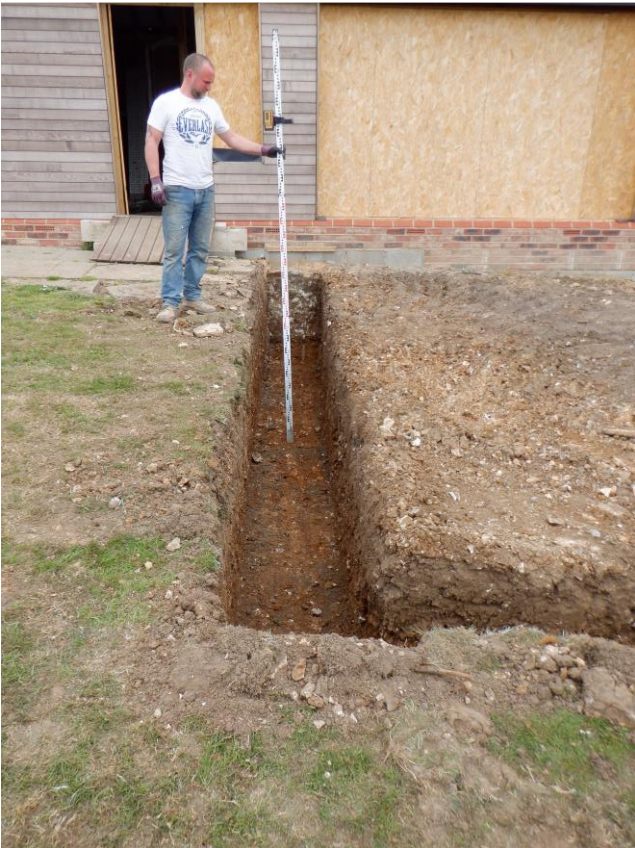
Plate 2. View of single storey extension foundations (looking N)
