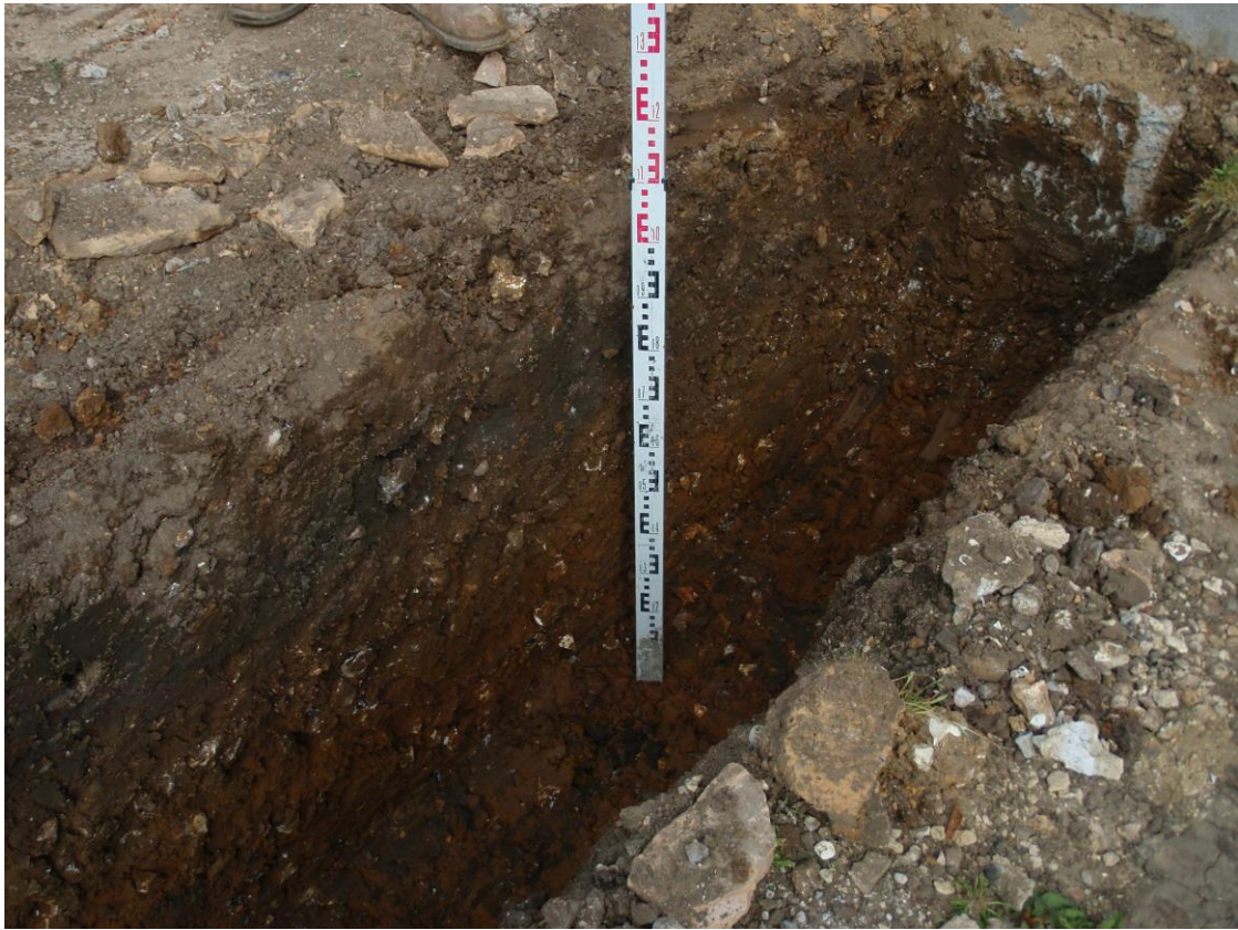
Plate 5. Garage foundation trenches (looking N)
